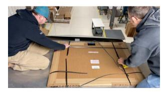
Once the straps are removed, the cardboard sandwiching the panel can be removed. Gently slide the bottom piece of cardboard out.
