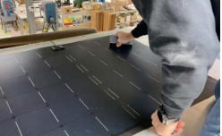
Slowly pull the double-release liner, and continue using the felt-tipped squeegee to work the panel down using the method described in 7.
