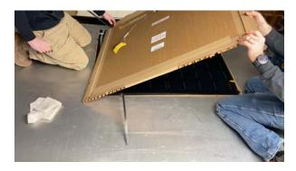
Slide the panel approximately into place. Now, you can remove the plastic clips holding the thin plastic.
