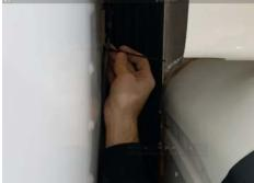
Affix the charge controller using included screws to a mechanically sound surface such as the side of a battery box or metal frame.
