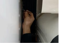
Affix the charge controller using included screws to a mechanically sound surface such as the side of a battery box or metal frame.
