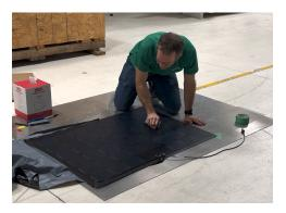
Slowly pull the double-release liner, and use the felt-tipped squeegee to work the panel down using the method described in 7.
