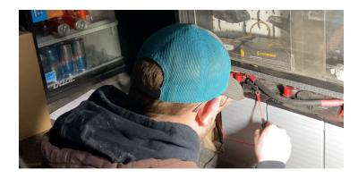
Measure the battery voltage to confirm 12V correct polarity, and reinstall the fuse. When the solar panel is exposed to sunlight, check the battery voltage. The battery voltage should be slightly higher depending on the amount of direct sunlight.
