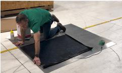
**THIS STEP IS CRITICAL**: To install the panel where intended, slowly pull the release liner, exposing 1-2 inches of the butyl adhesive. Ensure the panel is aligned as desired, and when ready, set the exposed butyl portion in the installation location. Use a plastic felt-edged squeegee to install the panel.
