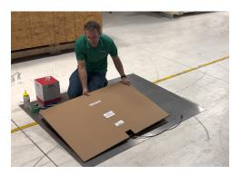
Slide the panel approximately into place. Now, you can remove the plastic clips holding the thin plastic.
