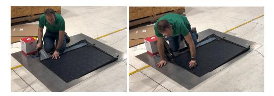
Slowly pull the double-release liner, and use the felt-tipped squeegee to work the panel down.
