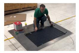
**THIS STEP IS CRITICAL**: To install the panel where intended, slowly pull the release liner, exposing 1-2 inches of the butyl adhesive. Ensure the panel is aligned as desired, and when ready, set the exposed butyl portion in the installation location. Use a plastic felt-edged squeegee to install the panel.
