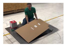
Slide the panel approximately into place. Now, you can remove the plastic clips holding the thin plastic.
