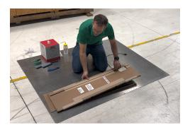
Slide the panel approximately into place. Now, you can remove the plastic clips holding the thin plastic.
