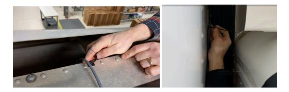
Remove the fuse in the wiring harness going from the charge controller to the battery.
