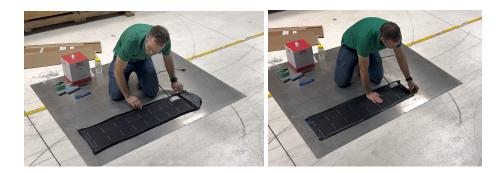
**THIS STEP IS CRITICAL**: To install the panel where intended, slowly pull the release liner, exposing 1-2 inches of the butyl adhesive. Ensure the panel is aligned as desired, and when ready, set the exposed butyl portion in the installation location. Use a plastic felt-edged squeegee to install the panel.
