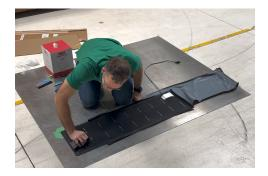
Slowly pull the double-release liner, and use the felt-tipped squeegee to work the panel down.
